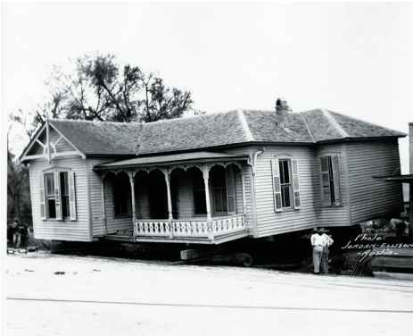
Destined for demolition, the O. Henry House was donated to the City of Austin, who relocated it to Brush Square to become a museum. (Credit: Jordan-Ellison Co, 1934. CO9584, Austin History Center, Austin Public Library)
