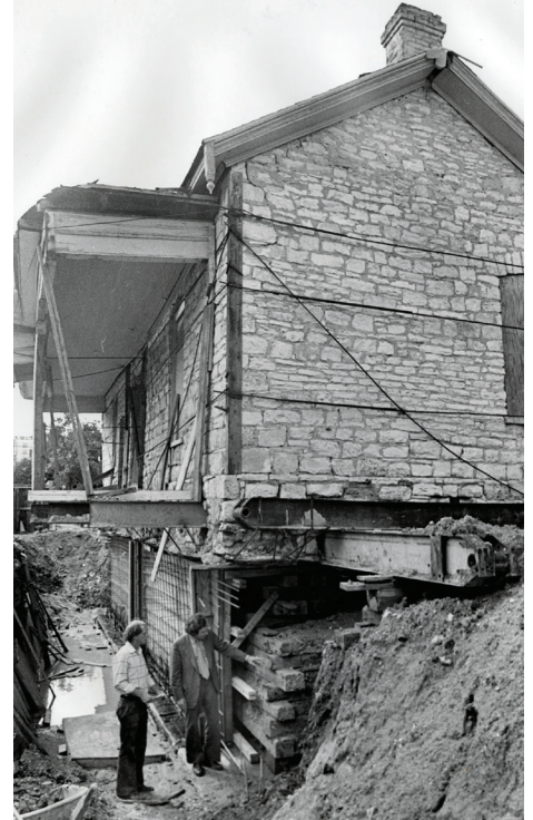
Following relocation to Symphony Square, a new foundation is designed to create a basement under the historic structure. (Credit: PICH-03729, Austin History Center, Austin Public Library)
