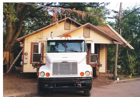
A house in East Austin is ready for transport. (Credit: Kathy Robinson)
